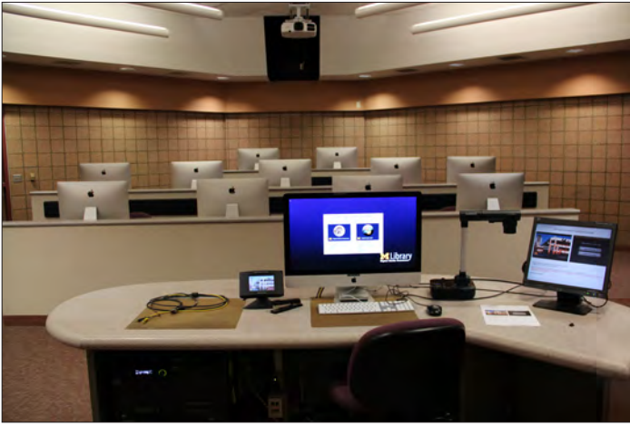
DC Multimedia Rooms IMG_6960
