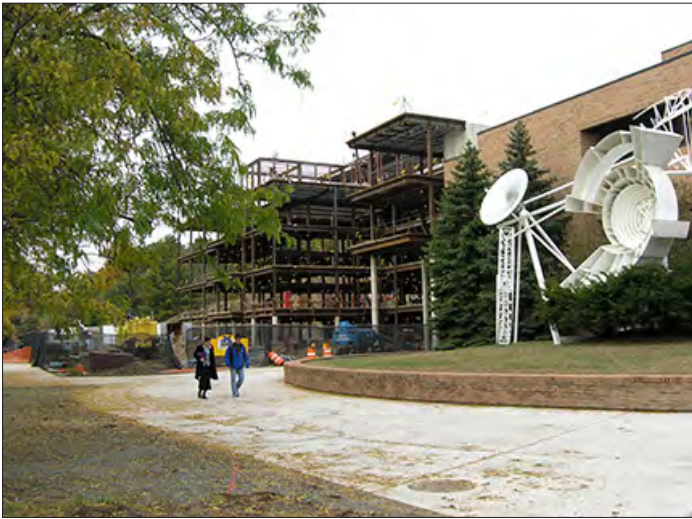
2004NewCSE Computer Science Building Construction (left)
