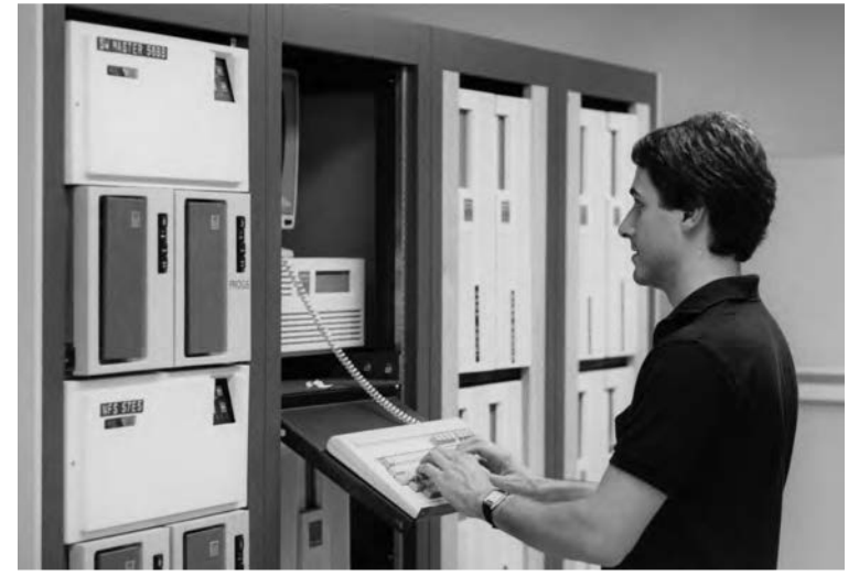
New machine room
